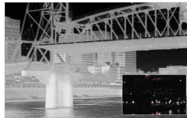
Thermal image of bridge structure at night and what the human sees (inset)
